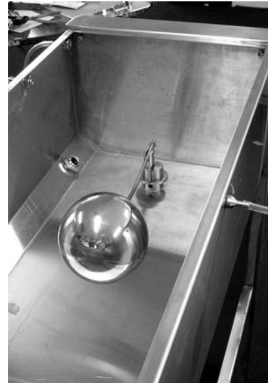
Fig 16. Float installed.
